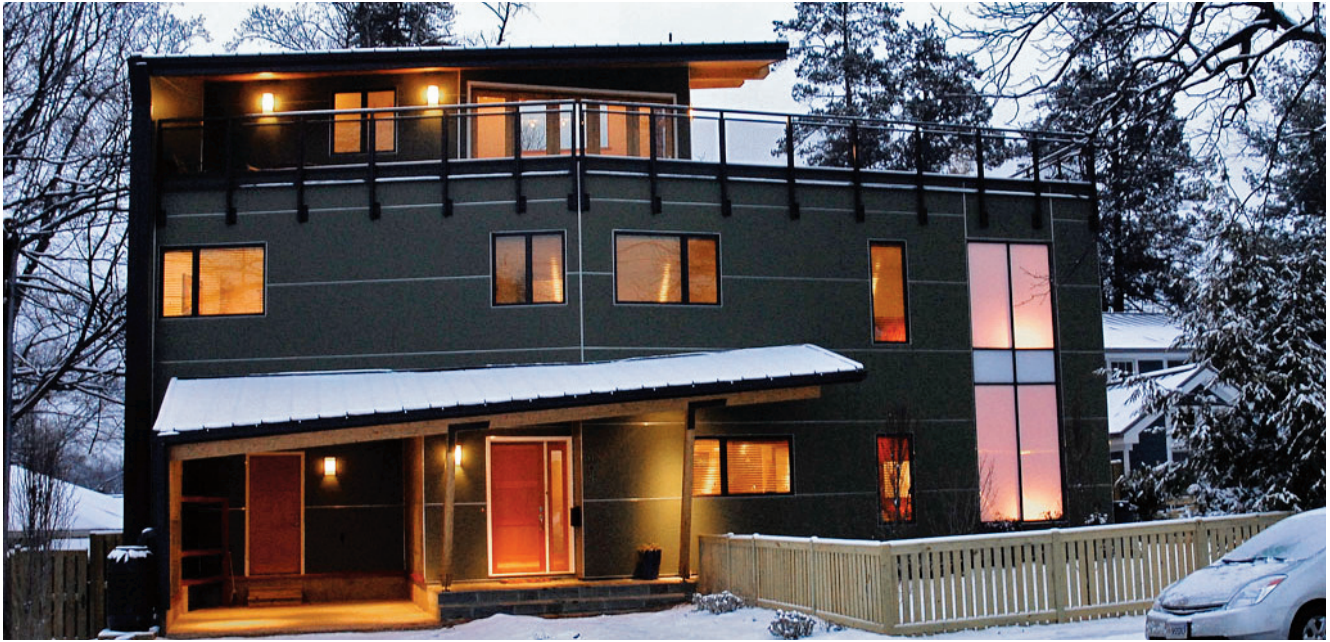
A UNIQUE TWO HOME PROJECT IN ARLINGTON, VIRGINIA COMBINING HISTORIC PRESERVATION AND ECO-MODERN DESIGN.
